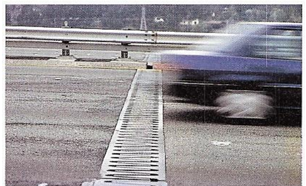
This gap in the roadway of a bridge is called an expansion joint; it allows the bridge to expand and contract. (Was this photo taken on a warm or a cold day?)
