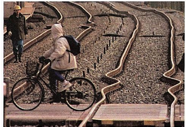
Thermal expansion. The extreme heat of a July day in Asbury Park, New Jersey, caused the buckling of these railroad tracks. ( Wide World Photos )
